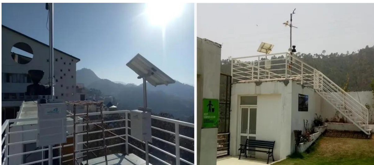
Automatic weather station installed to monitor changes in weather.
