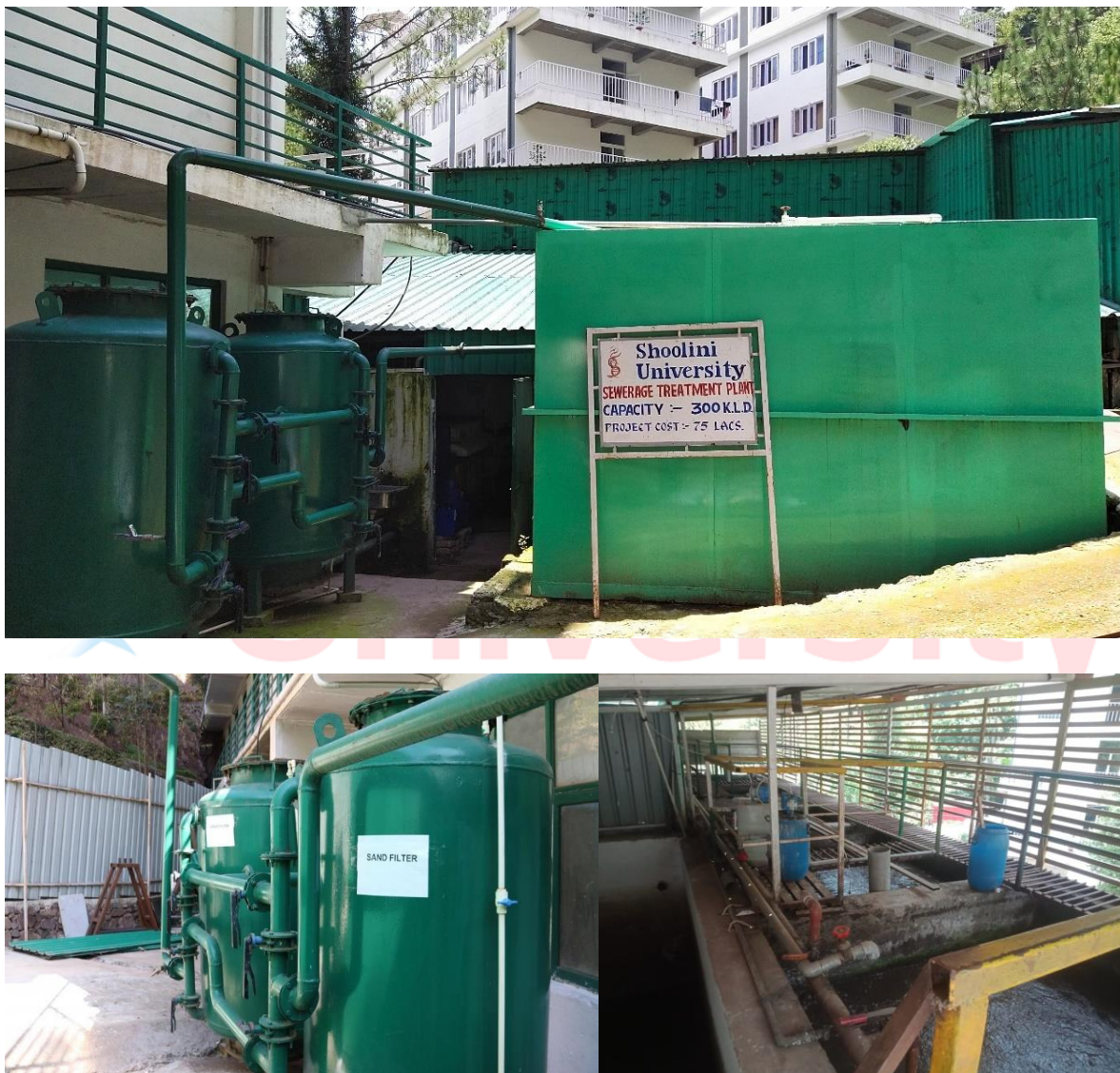
Figure 5: Sewage treatment plant
