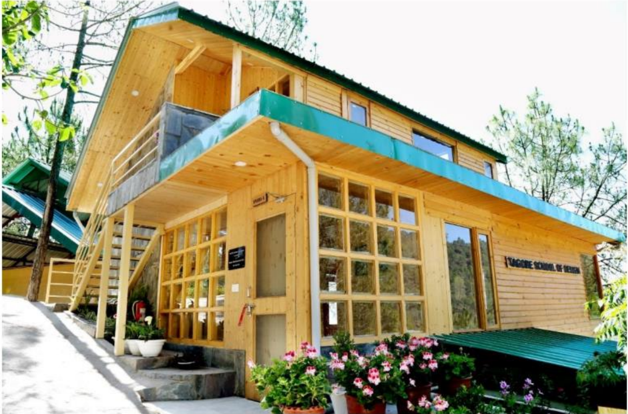
Side view of School of Design Sustainable Building
